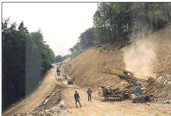
Example: Drilling work using a crawler-mounted drilling device.
