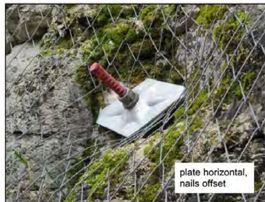
THE FINISHED TECCO® SYSTEM LAYED AND TENSIONED
